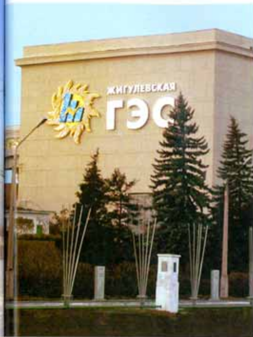
The solar "energy emblem," which sits 42 ft. high, comprises steel tubing, a Dibond® base layer and stainless-steel cladding. Double-halo blue neon and exposed, yellow neon illuminate the emblem and channel letters. The tubes incorporate argon and K4 (a neon and argon mix), which endures cold climates well.
